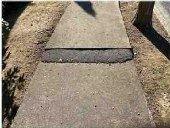
69. Outside 10 Kimberley Grove
