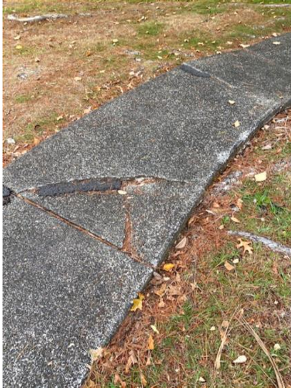
Opposite No 30 Kingfisher Grove. The link from one side of Kingfisher to the other.
